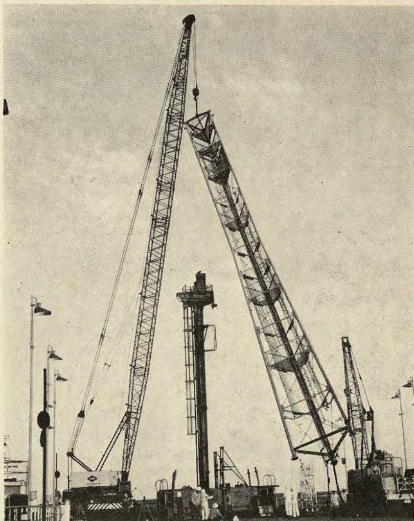
This picture shows one stage of erection of a 100 ft. high umbilical mast at the Eldo launching site at Lake Hart. Most of the work was done using a Lima crane capable of lifting a load of 45 tons. It can reach a height of 160 ft. and is one of the largest fully mobile cranes in South Australia. The crane is operated by the Engineering Group, Woomera.
