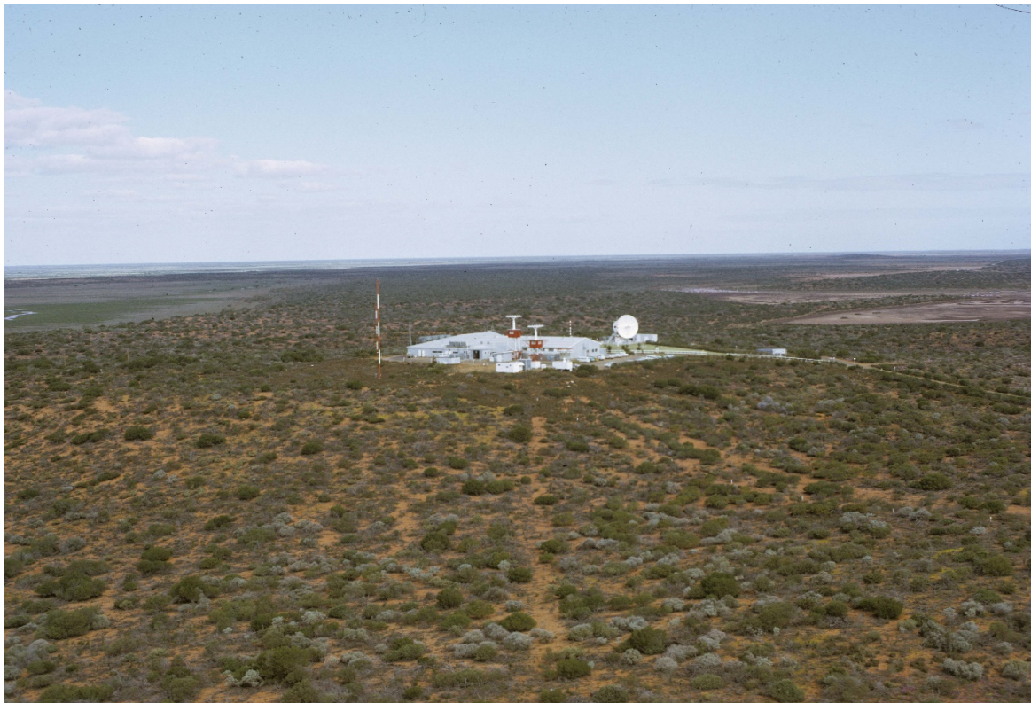
Looking south east, from the top of a USB calibration tower toward the main tracking station building, the Telemetry and Control building, T&C.
