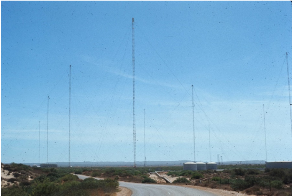
The Transmission aerials at Exmouth
