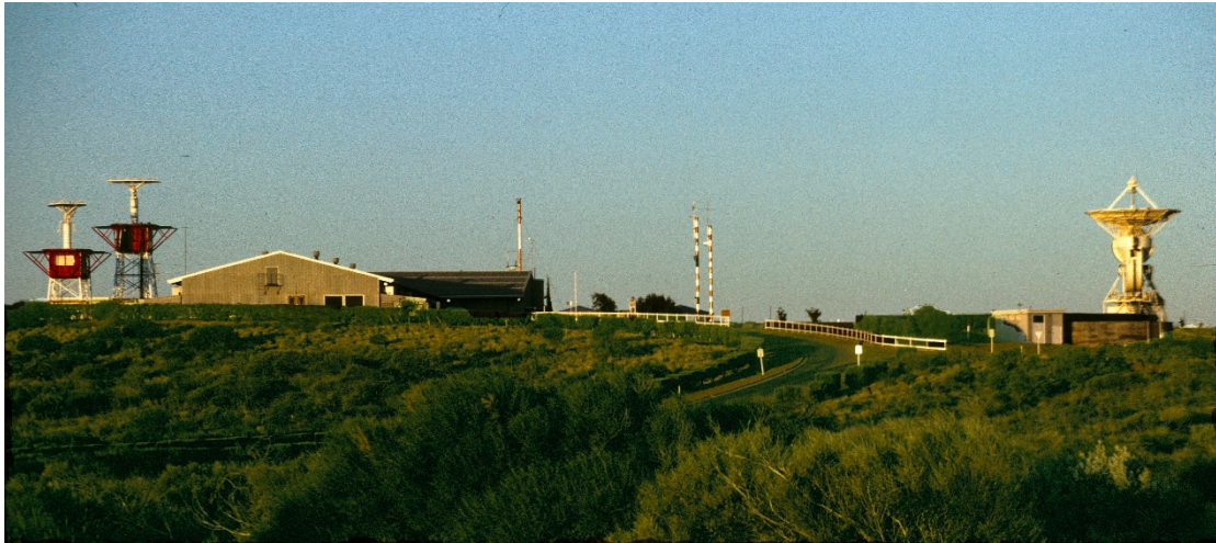
View of the T&C building from SPAN, USB antenna on right
