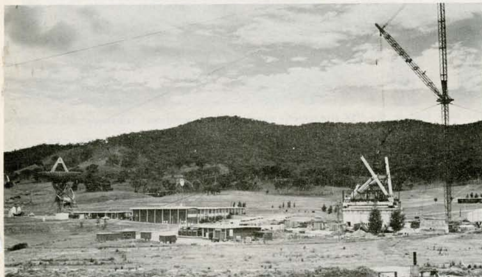
The Tidbinbilla Deep Space Communications Complex (TDSCC) comprising: right, DSS42A (DSS43 when operational) 64-meter antenna (210 ft); left, DSS42 26-meter antenna (85 ft); microwave link dish and tower to HSK at center; and the MSFN wing is in the blank walled building in the center, added to the existing DSN operations building.
