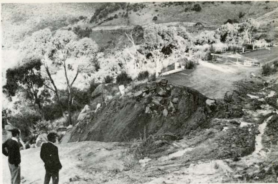
The main road to the HSK site recently caved in due to persistent rainstorms and flooding throughout the area.
