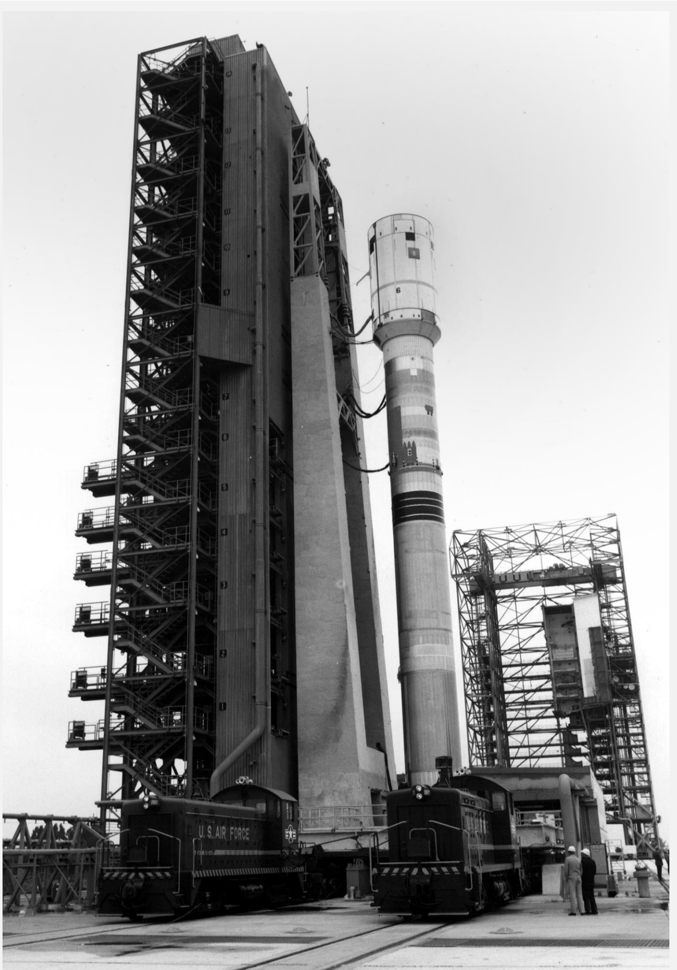
The Titan-3E, Centaur-D1T and Star-3E stages are stacked and moved to the assembly stand in preparation for the arrival of the payload fairing containing the Voyager 1 spacecraft. Image: NASA/KSC
