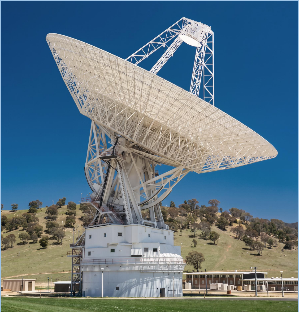
Deep Space Station 43 at Tidbinbilla in its original 64-metre (210 foot) configuration. Image: CDSCC Archive
