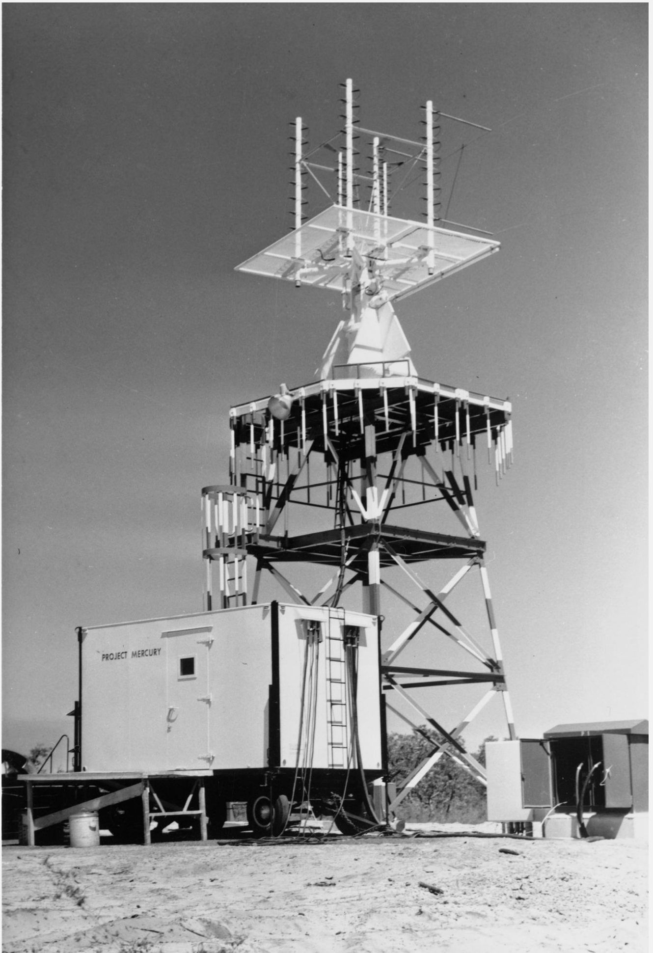
The north-most of the Acquisition Aid antennas adjacent to the Telemetry and Control Building.
