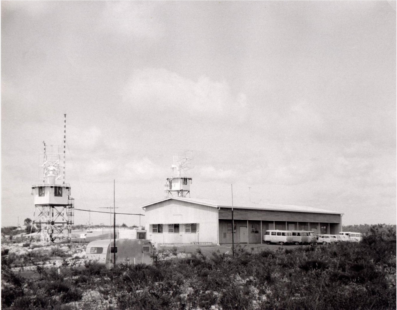
The Telemetry and Control (T&C) building with the security caravan in the foreground. Behind the building are the Acquisition Aid (Acq Aid) quad helix antennas. Photo: Hamish Lindsay
