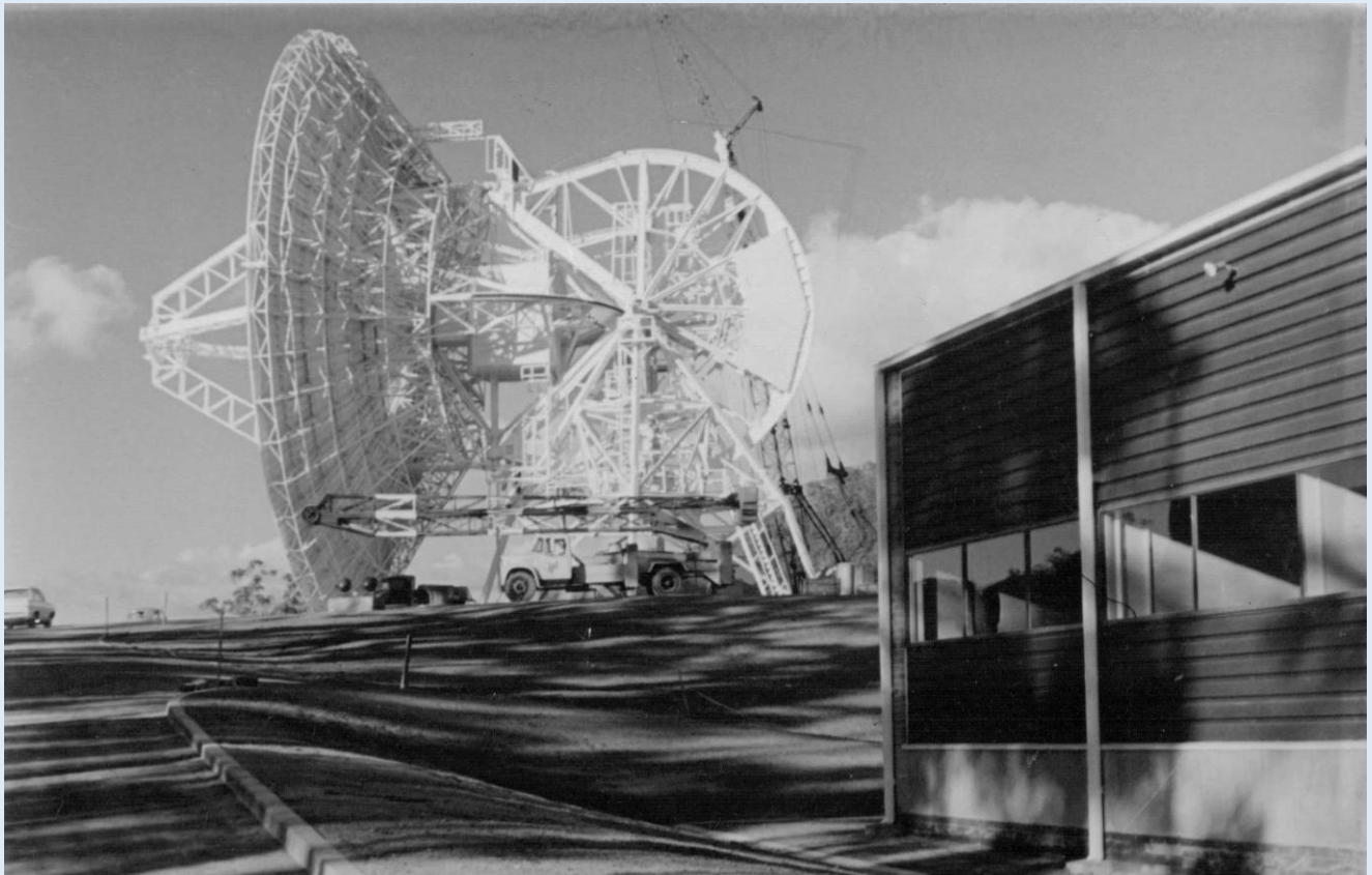
The Honeysuckle antenna during construction. Photo: Frank Barrow
