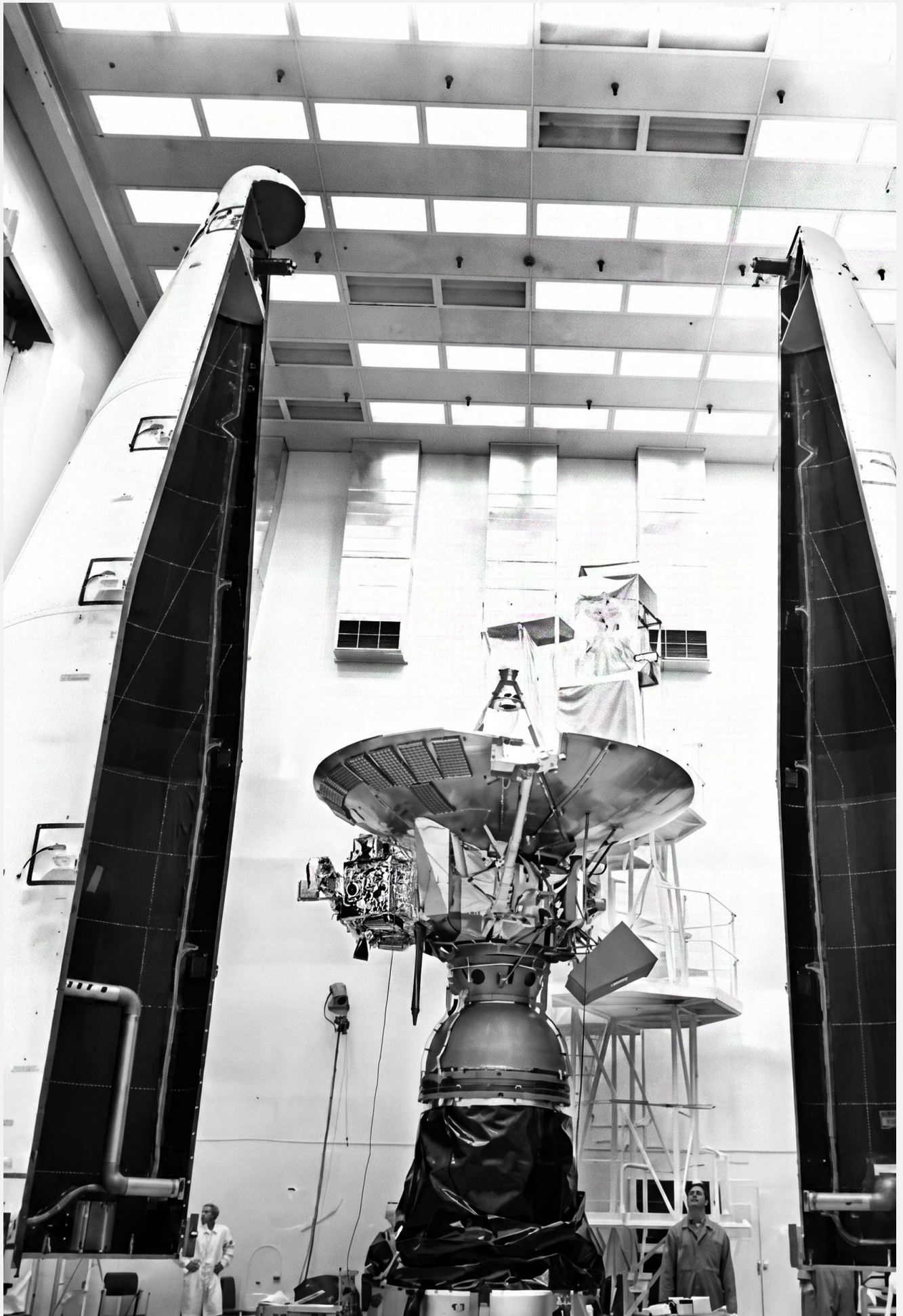
Pioneer 10 nearly ready for encapsulation in its payload fairing. Image: NASA/KSC
