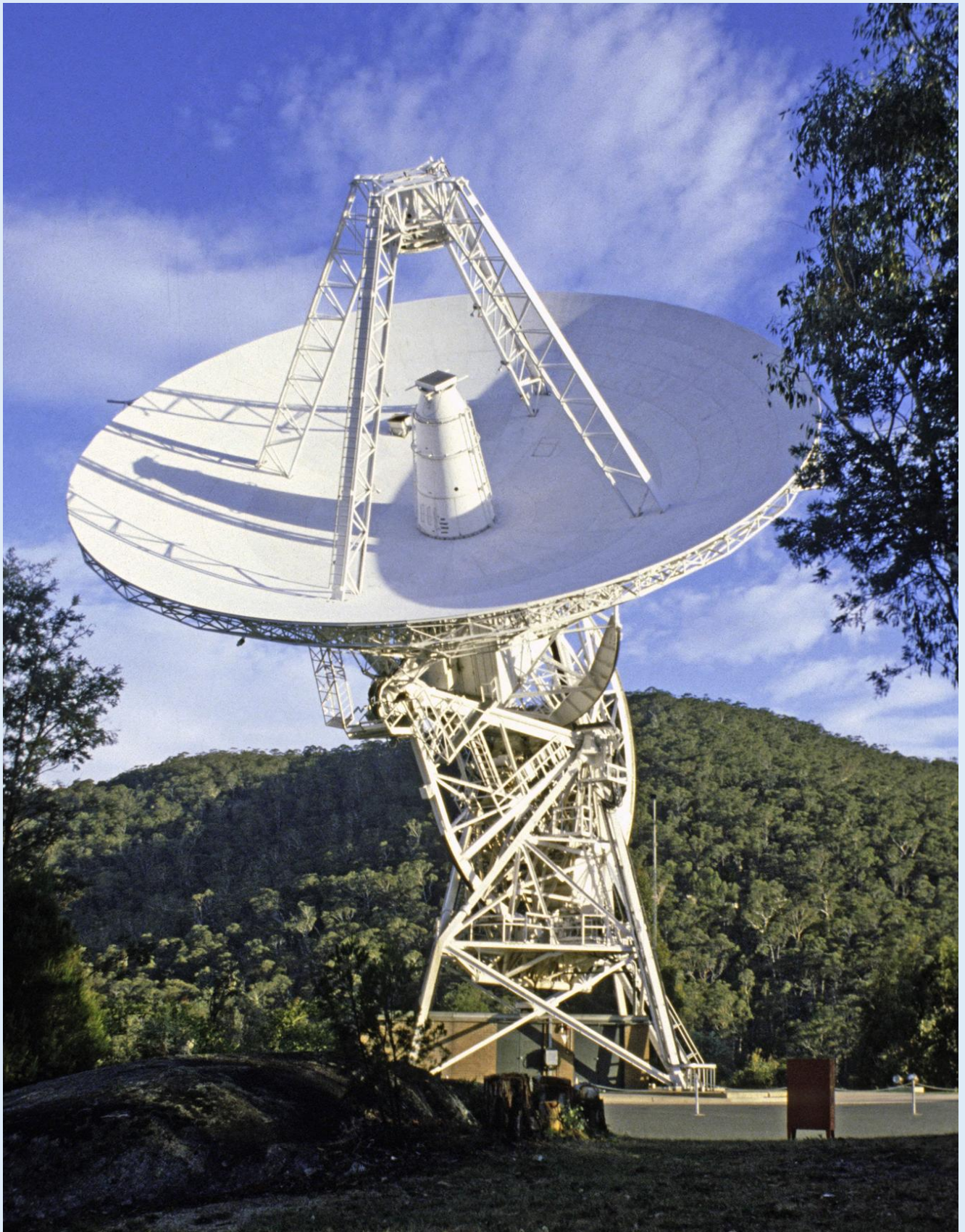
Deep Space Station 44 at the Honeysuckle Creek Tracking Station.
