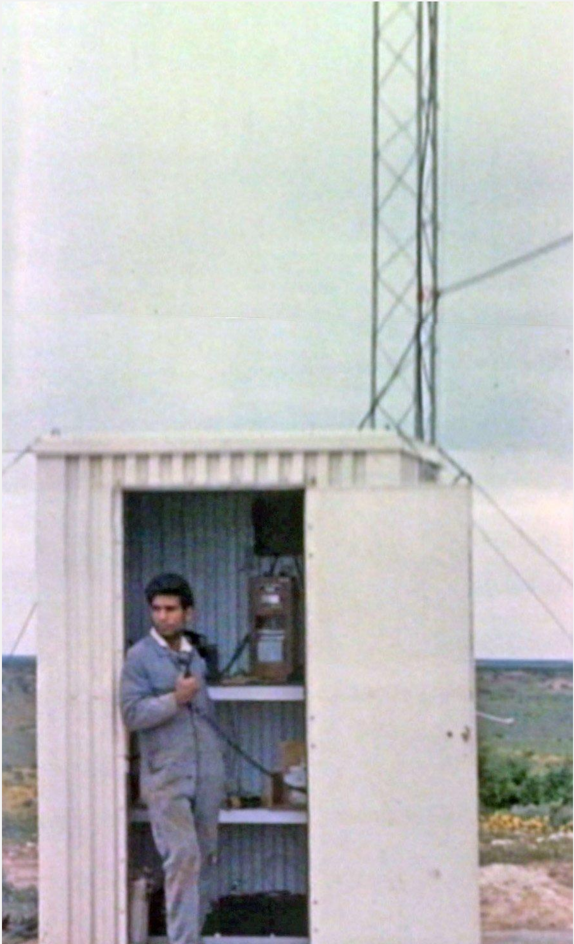
A closeup of the relay hut at Yaringah Hills. Image: Dept. of Supply film
