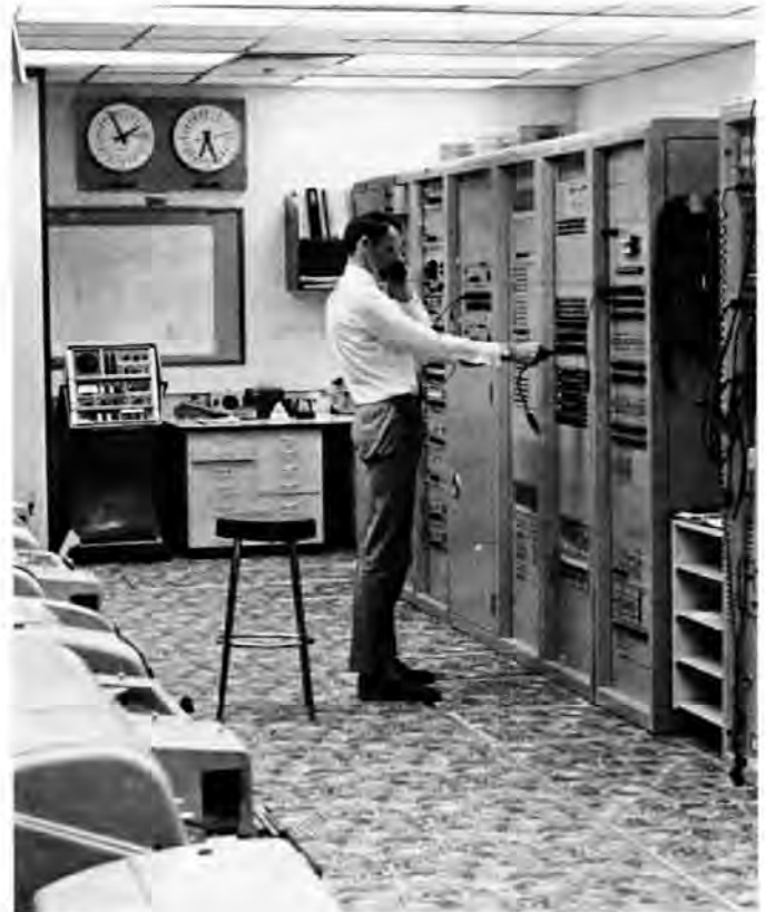
Communications room at the Woomera Deep Space Station.
