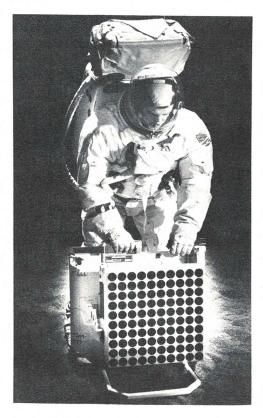
An engineer is shown demonstrating the emplacement of a Laser Ranging Retro—Reflector, one of two experiments in the Early Apollo Scientific Experiments Payload, for deployment on the first lunar landing.
